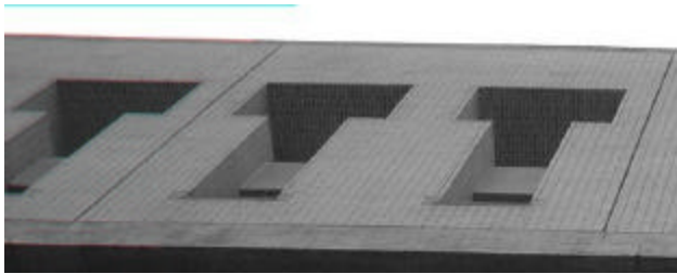
Figure 4 Part of the decentering distortion rectified image.
