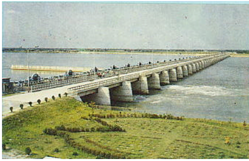
Fig. 2 The Barrage constructed in Teesta R.
