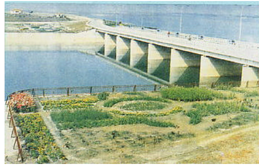
Fig. 4 Canal head works (110m in length , maximum intake flow: 280 m 3 /sec)
