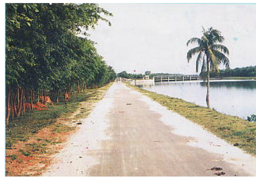
Fig. 5 Main canal in project area and inspection road in the left bank
