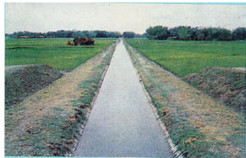
Fig. 6 A lined tertiary canal and paddy fields planted HYV rice.
