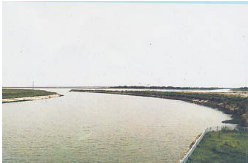
Fig.3 Silt trap pond covering 45 ha adjacent to intake gate of main canal
