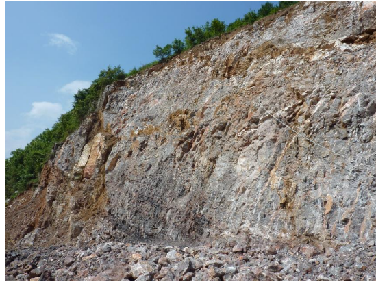
Figure 12: Drilling results for a deduced broken bedrock band.
