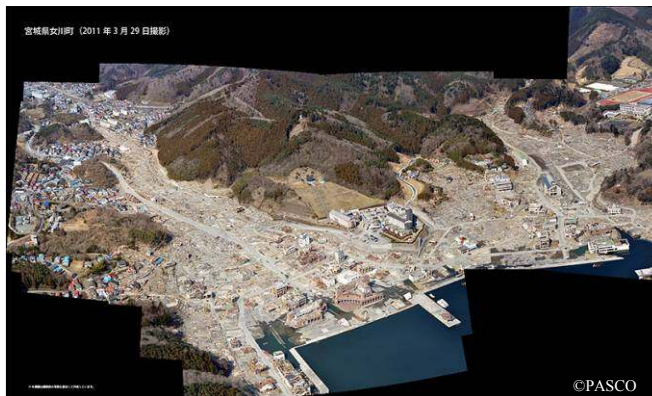
Fig.5 Panoramic oblique photo (Onagawa city, Miyagi Pref.)
