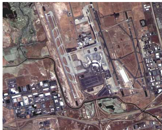
Fig.15 pan-sharpened 2.5-metre GSD multispectral image of Salt Lake City airport ((© NASRDA 2011)
