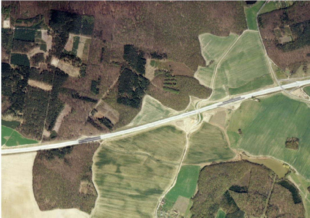
Figure 5: A problematic part of highway D11
