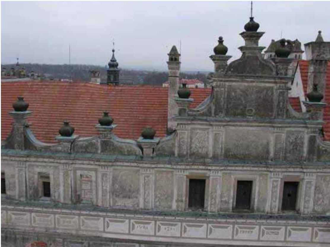
Figure 3 : Images from reconnaissance flight taken from hexa-copter over Litomyšl castle in the Czech Republic; no scaffolding or pull platform was needed
