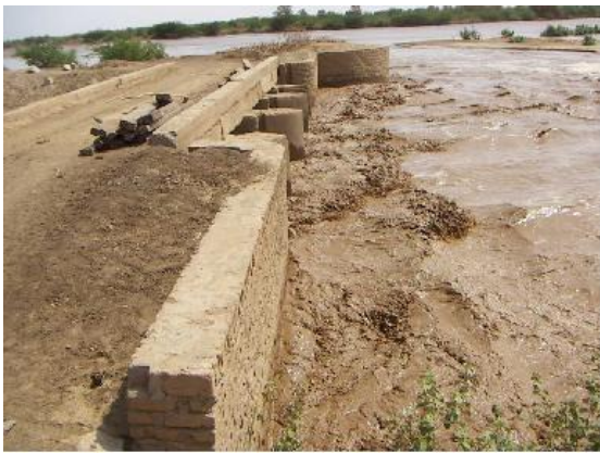
Fig. 4 Sluice gate from Gash River
