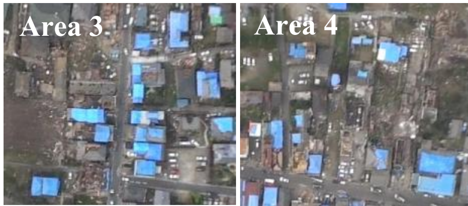
Figure 8 Target areas of heavy-damage in Figure 4.
