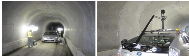
Fig. 7 Tunnel wall inspection by IMS3
