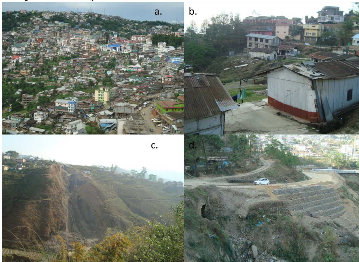
Figure 5. a). Portion of the study area- note the closely constructed heavy concrete construction on unstable slope. b). Affected buildings in Ward no.1 of the study area. c). Landslide with an approximate length of 150 m in Ward no. 6. d). Landslide at Asian Highway (AH) 1 in Ward no. 18.
