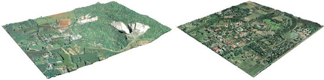
Figure 5 3D city model over rural (top) and urban (bottom) regions created by using point cloud and aerial image of MOST dataset
