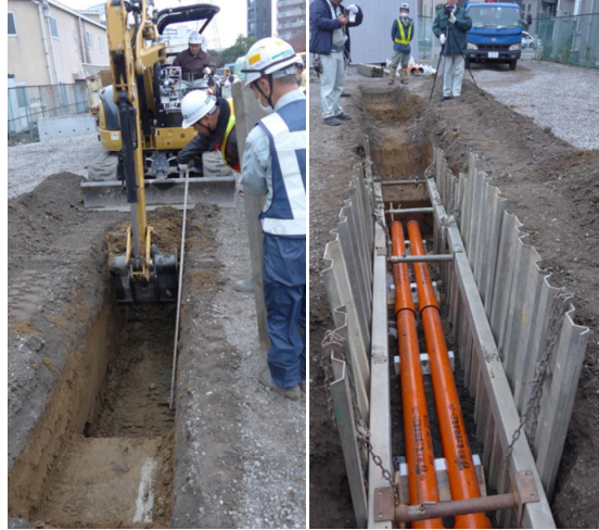
Figure 6. Simulated construction environment
