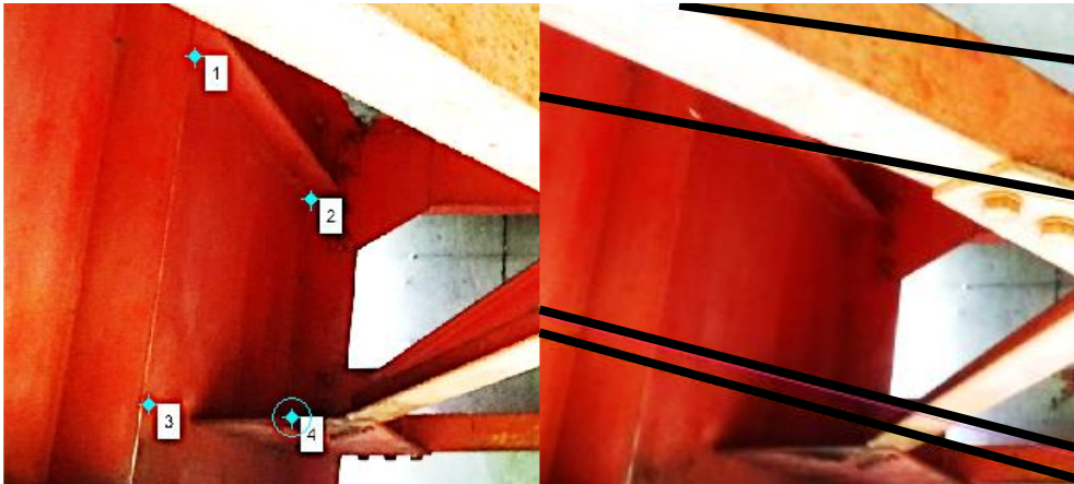
Figure 8. Estimated epipolar lines (Left: base image, right: reference image)
