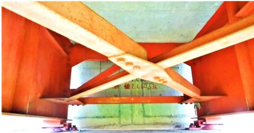
Figure 5. Measured object (metal girder bridge)
