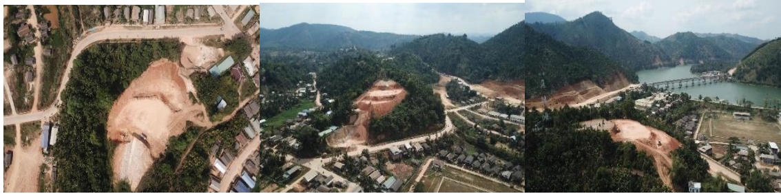
Plate 3.2. New construction sites in Tanintharyi
