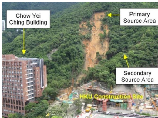
2008 Landslide behind HKU
