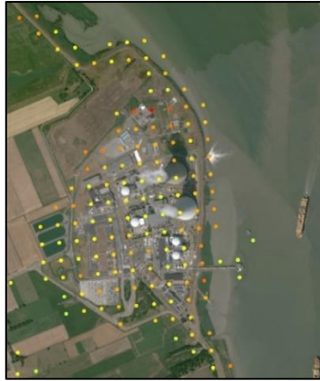
Figure 9 Overlay of EGMS Level 3 Ortho product covering the Doel nuclear power plant (extracted from https://egms.land.copernicus.eu/ produced with funding by the European Union)
