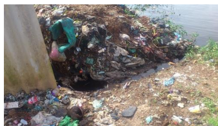
Figure 5: Direct leachate to the channel
